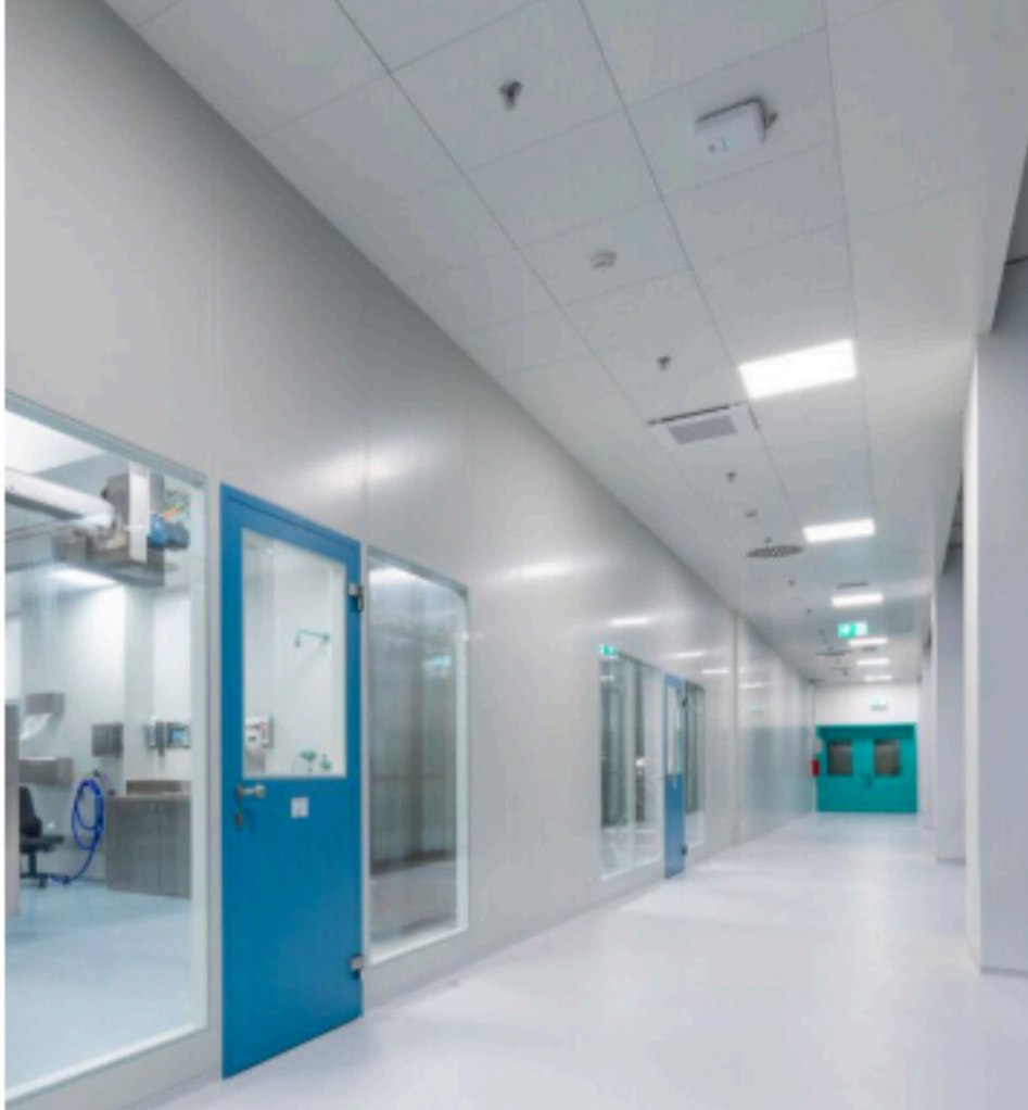
Clamping cassette ceilings are suspended metal ceilings that cannot be walked on. Lights and air outlets can be integrated into the system and lay almost flush with the surface (Source: Jens Distelberg)
