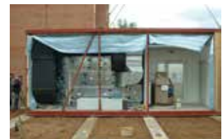
Positioning of the first module
