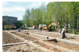
Preparation of the strip foundation on-site
